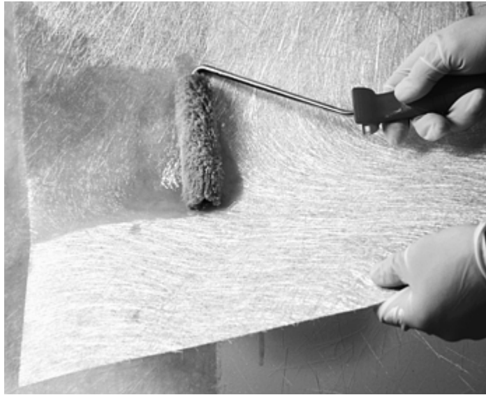
Fig. 7 Application of resin and chopped strand mat
