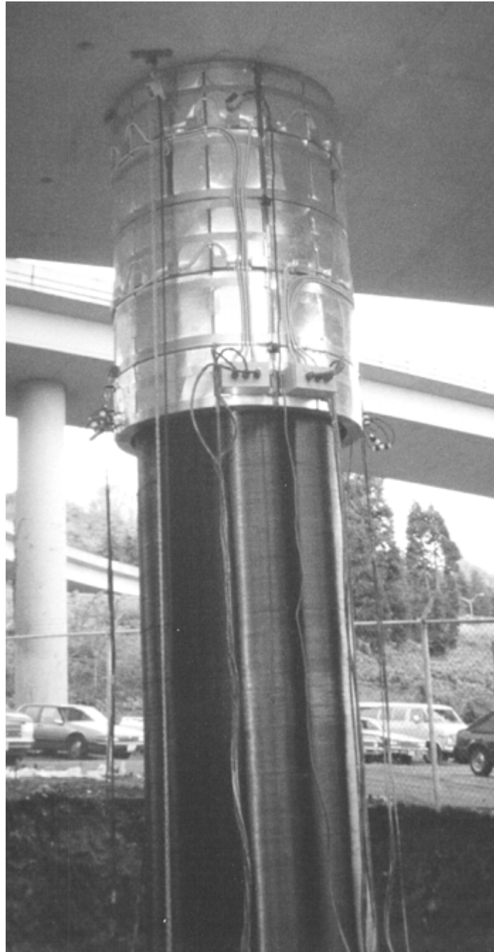
Fig. 5 Portable oven (Robo-Curing System) for curing columns wound from prepreg carbon tows. Courtesy of XXsys Technologies, Inc.
