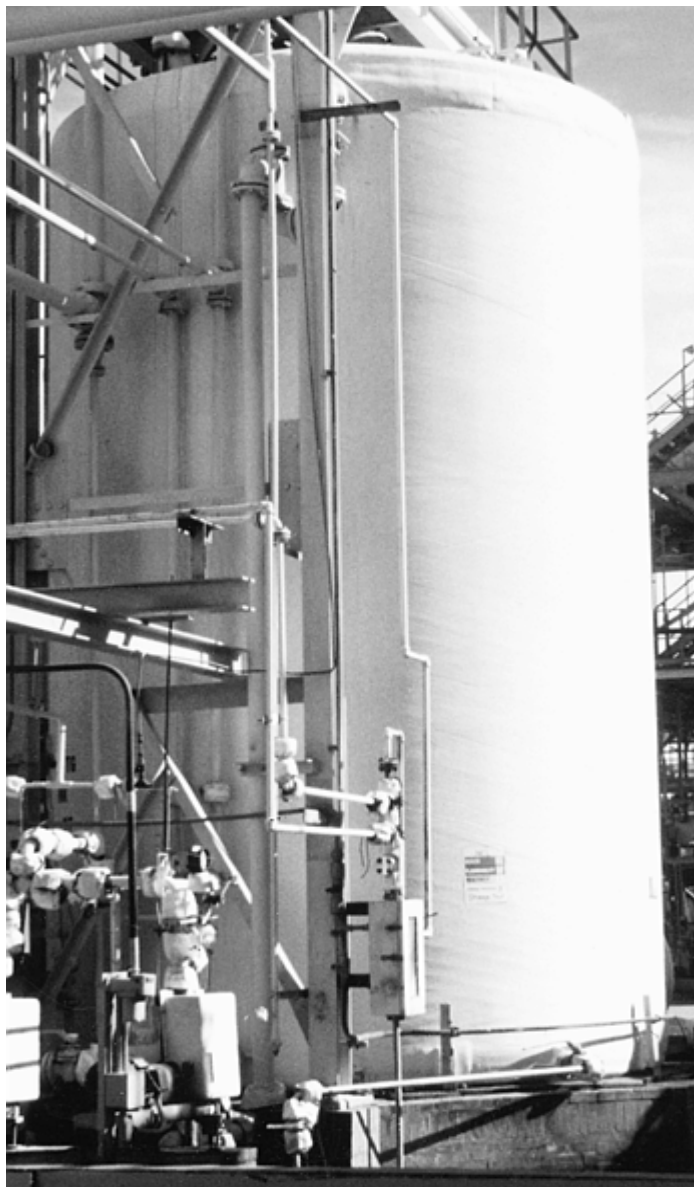
Fig. 3 Open-molded composite chemical storage tank. Courtesy of OxyChem
