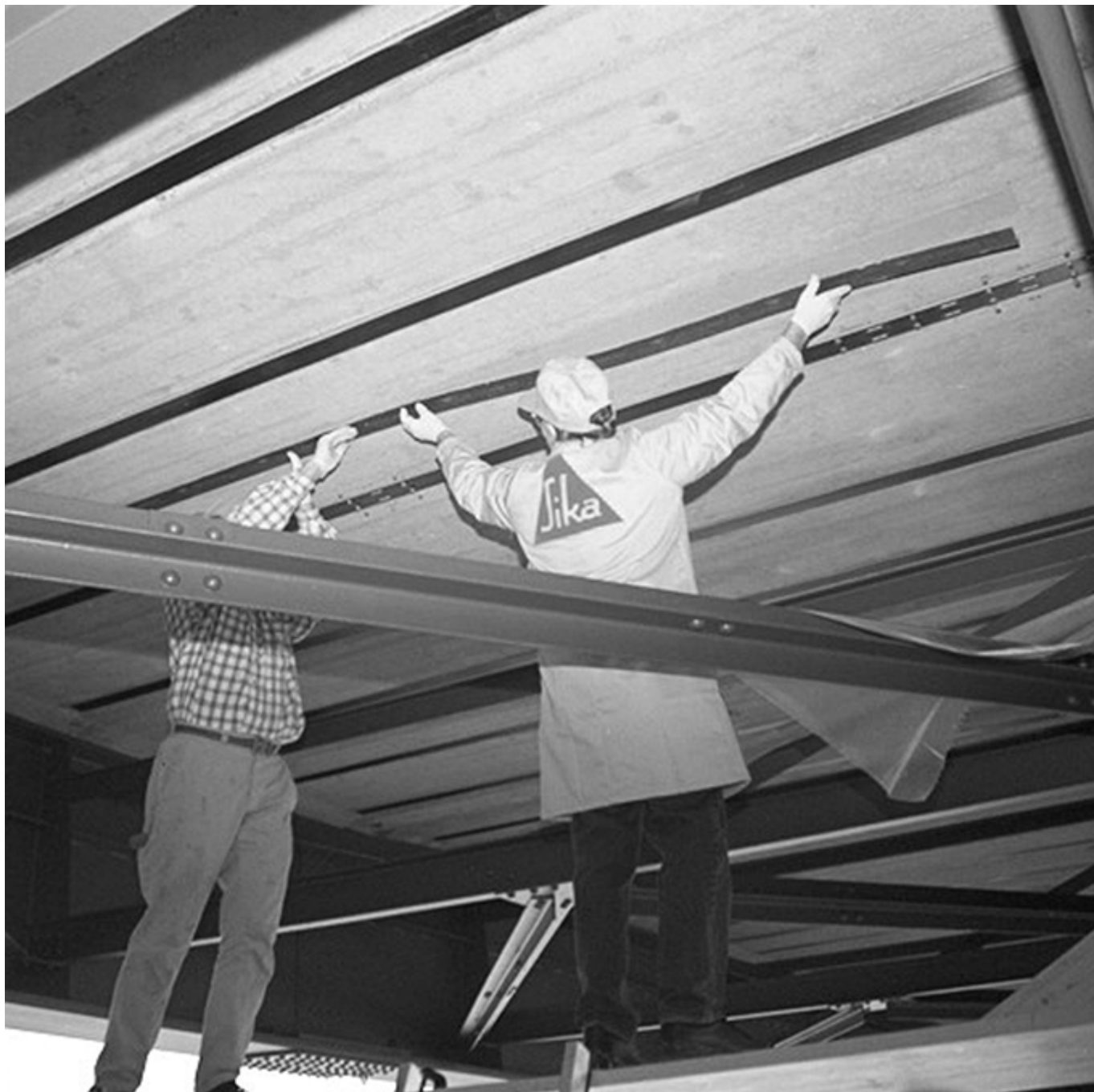
Fig. 2 Application of shop-manufactured carbon composite plates to the underside of a bridge deck
