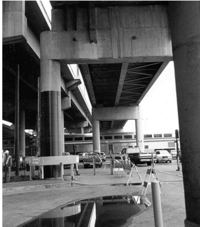
Fig. 3 Columns on the Santa Monica viaduct wrapped with carbon/epoxy prepreg
