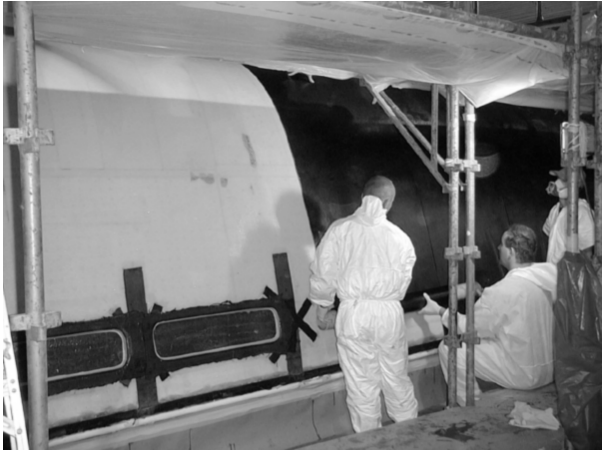
Fig. 9 Laminating a male molded hull
